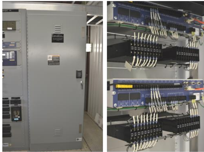
Figure 3. Entergy Secure Phasor Cabinet, Front View (left) and Interior View (right)
