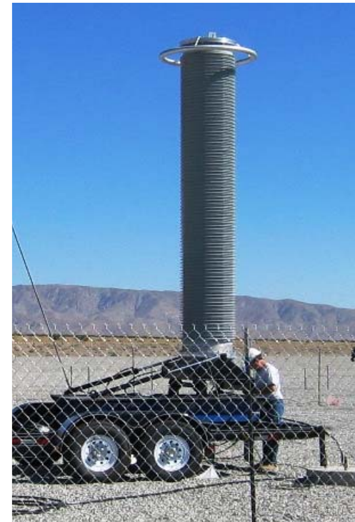
550 kV class testing for harmonics (Bandwidth 20 kHz)
