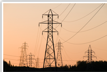
735 kV lines near the 5 616MW Robert-Bourassa generating station
