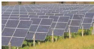
Solar farm to supply common areas such as a water treatment plant, community center and swimming pool
