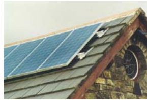
Rooftop solar for serving as Distributed Generation (DG) for each home
