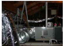
High efficiency HVAC systems with central Indoor Air Quality (IAQ) systems
