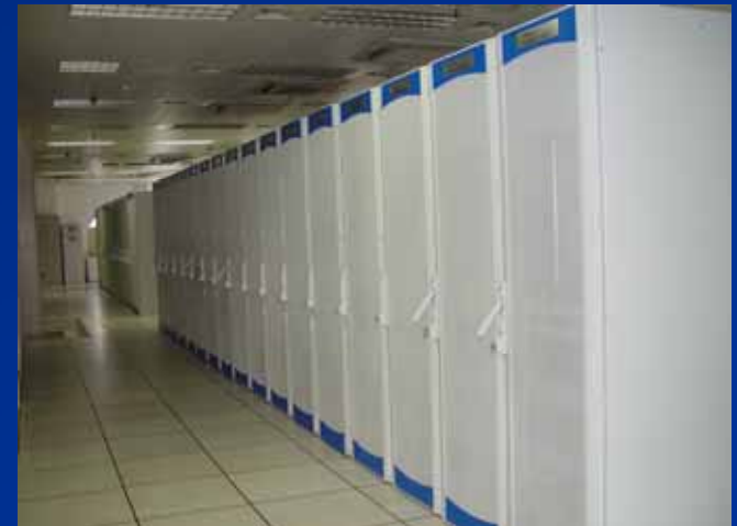
Master station computer Room
