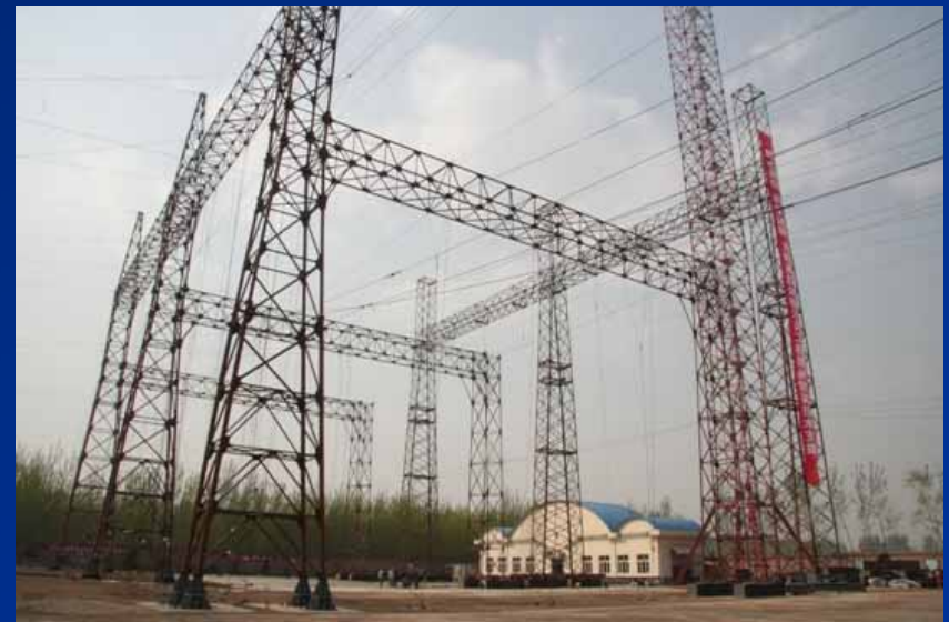
1,000kV AC Model Pole & Tower Test
