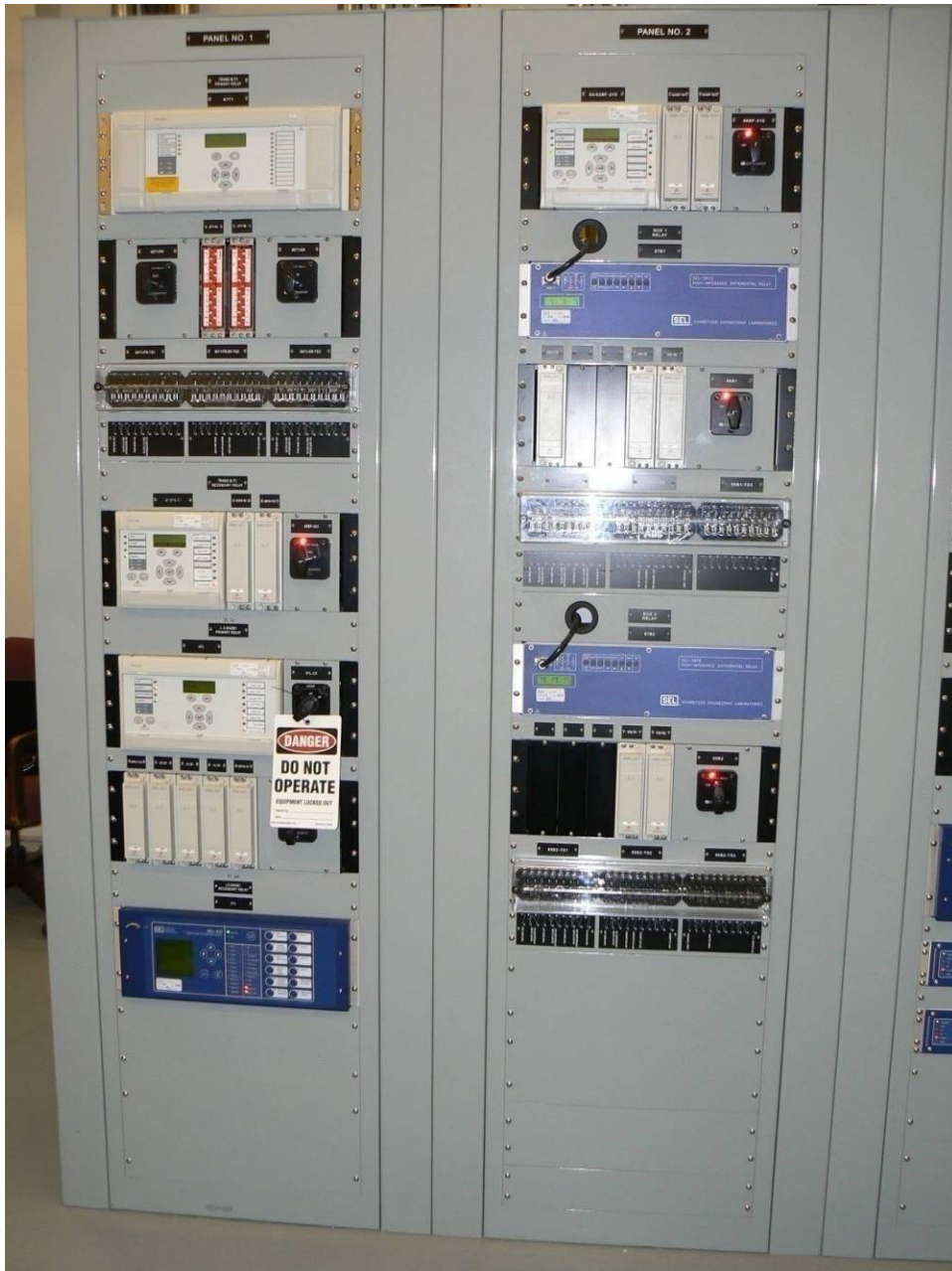
Long Bay Substation Typical Relay Panel
