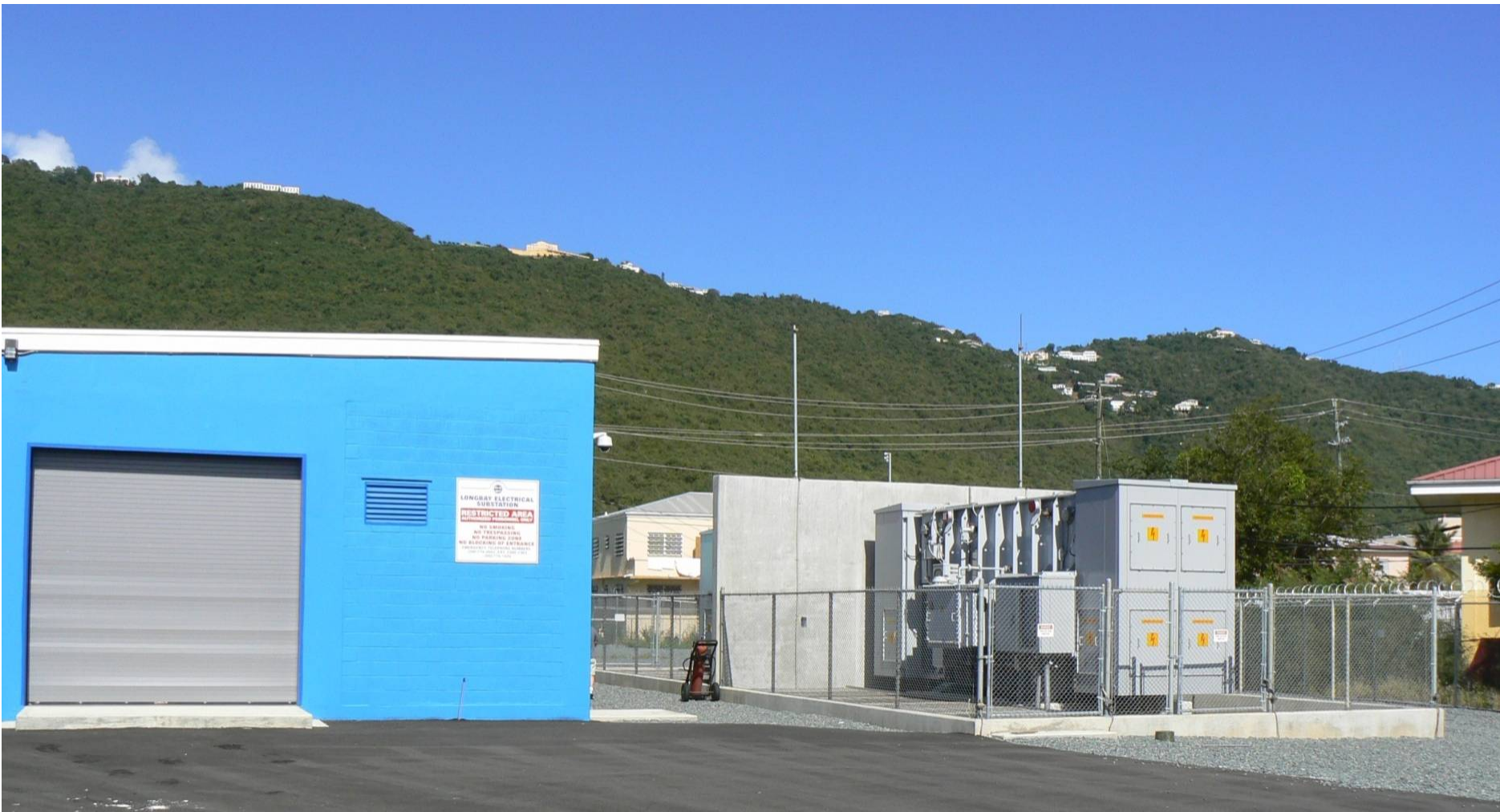
Long Bay Substation
