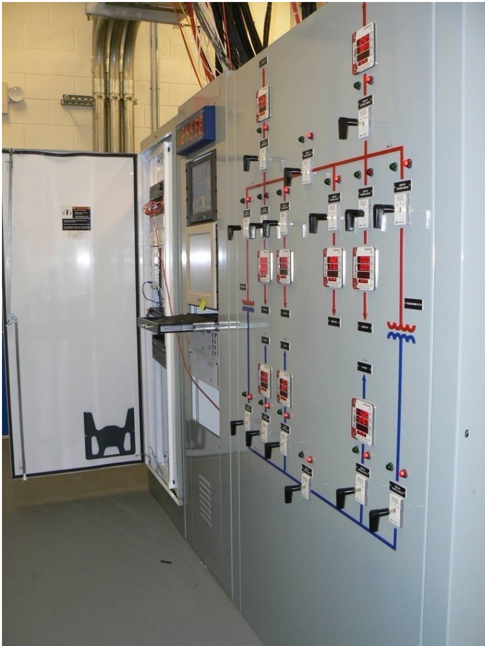
Long Bay Substation Control Room
