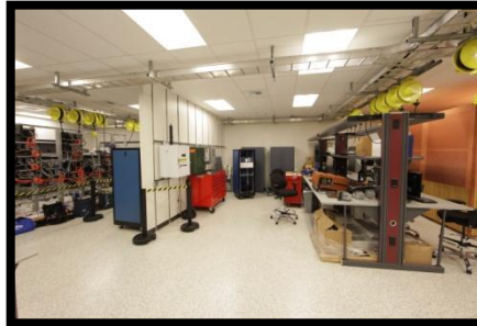
Distribution Automation Lab
